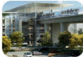
Consolidated Rent-a-Car Facility (ConRac)
