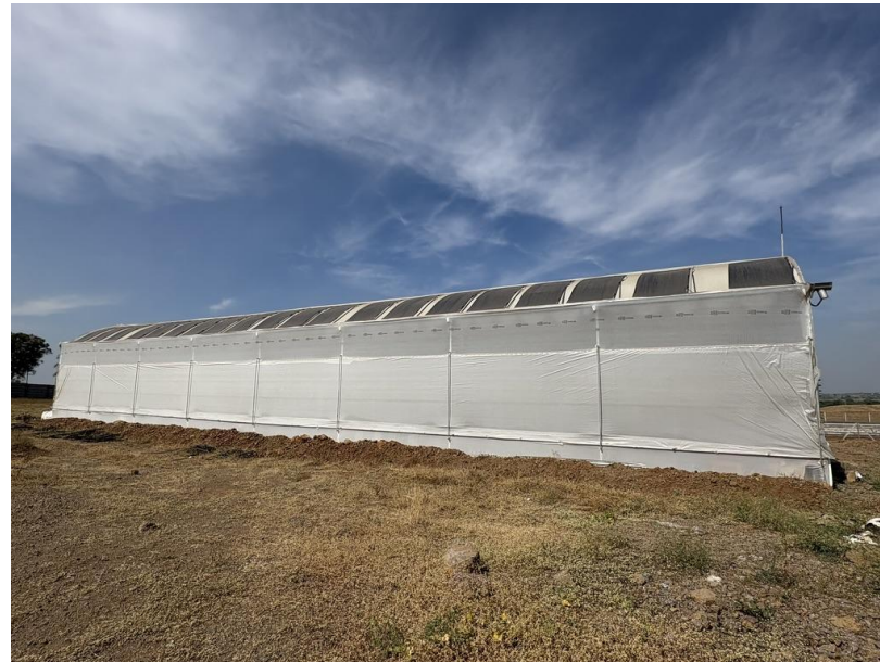
Greenhouse with solar panels to run fans
